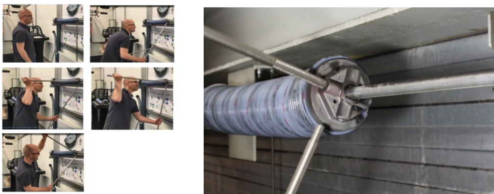
Figure 1 Left: Manual tensioning of an overhead door spring. Right: detail on working with bars/rods.
